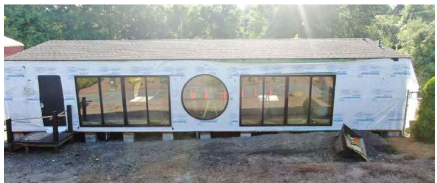
Drone photo from Armadas Exterior looking into the new building.
