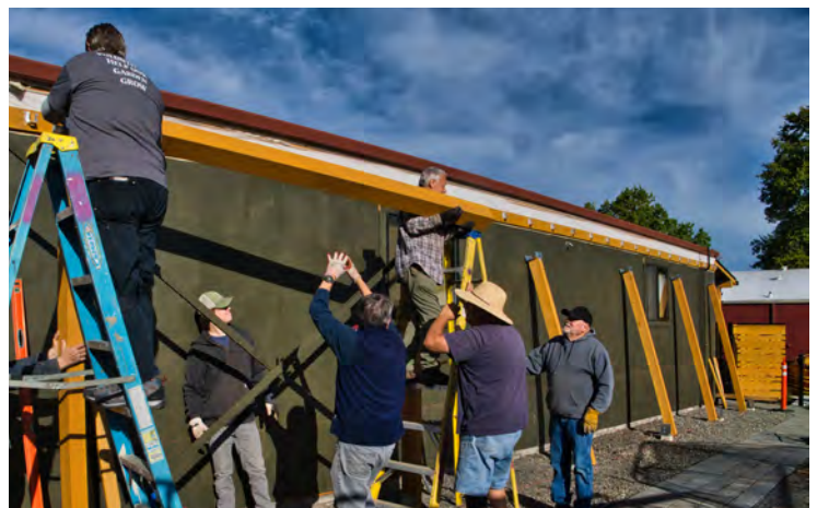
Volunteers hoisting the beam into position for the overhang.
