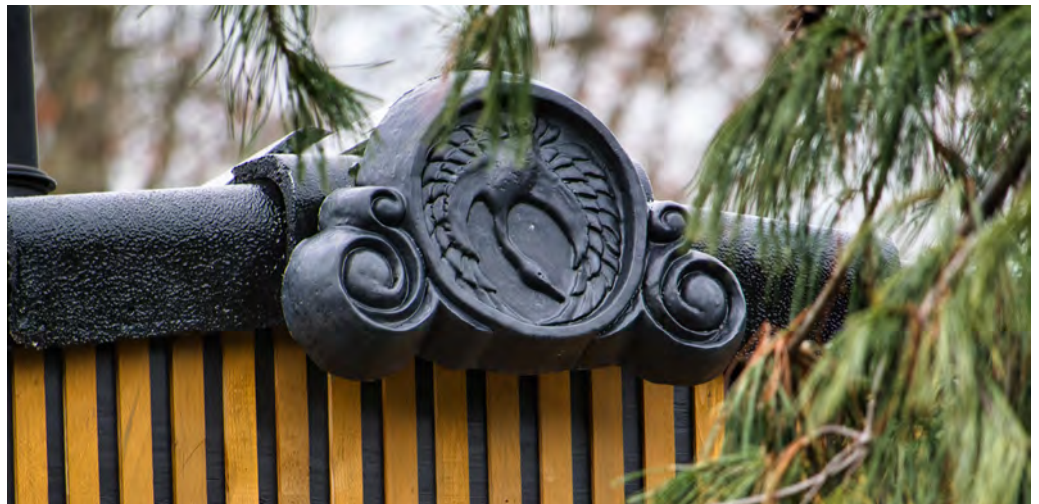
The onigawara on the roof of the Kyoudou Center.
