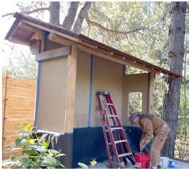
Chuck Page applying the final plaster coat.
