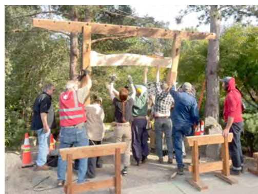
The hoisting of the structure.
