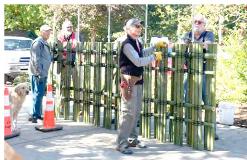
Volunteers carrying the heavy teppo-gaki panel to be installed.
